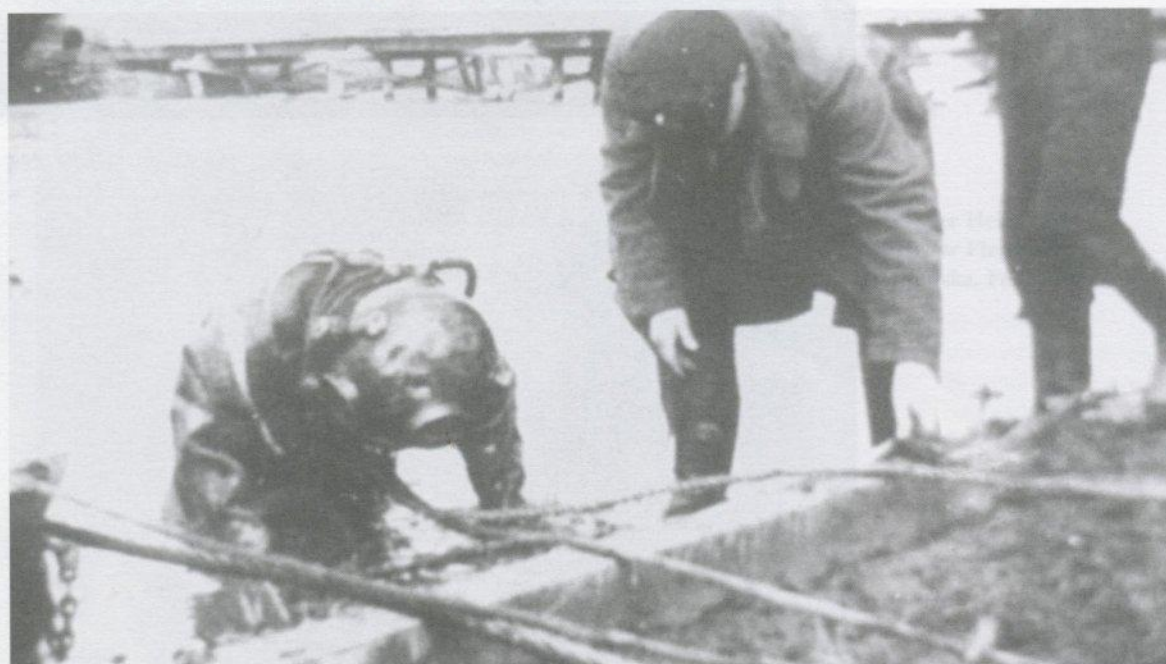
Divers connected the recovery cable of the prime mover to the sunken tank. The Mius bridge is in the background.
