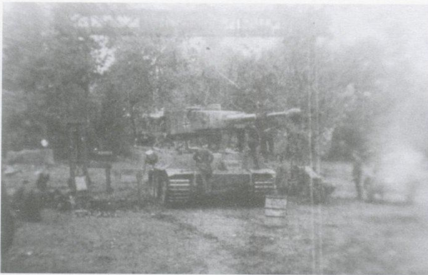
A Tiger turret is suspended from a portal crane in order to exchange or repair an important component. The operation has been skillfully camouflaged against observation from the air.
